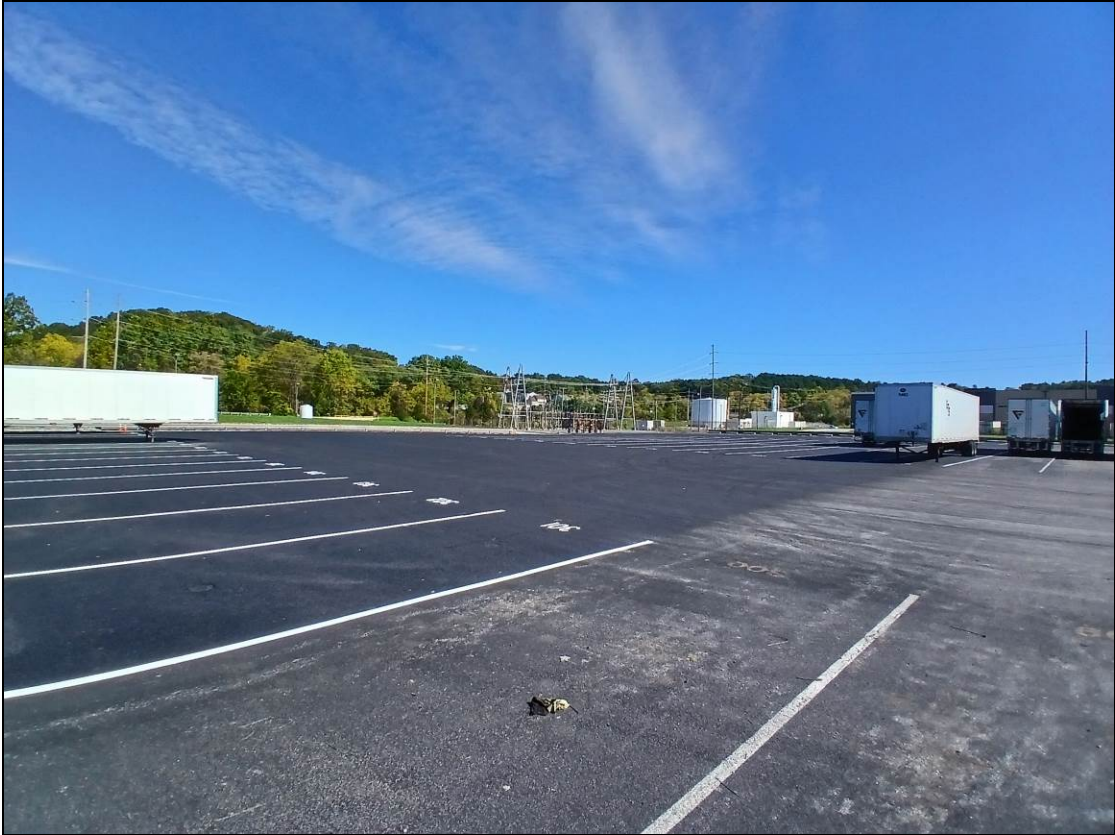
Photo 6: Photo looking northeast at northern fourth of WPL where asphalt seal coat was applied.
